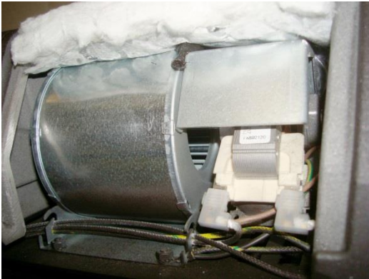
Figure No.15 - Access to fans
